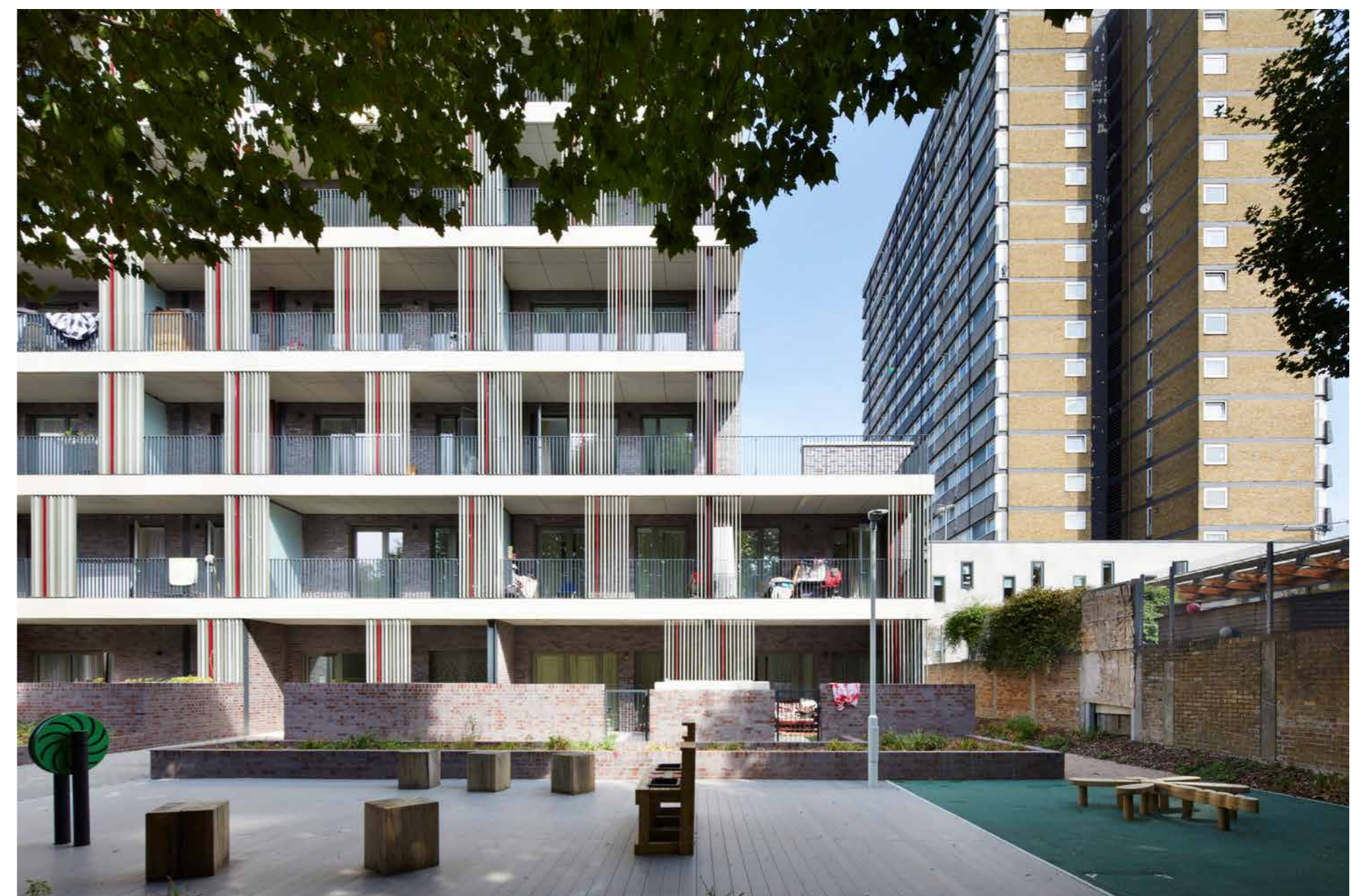
Rear view of Block A - now called Flats 1-38, 14-16 Wrotham Road - which comprises 38 council homes and completed in April 2018
