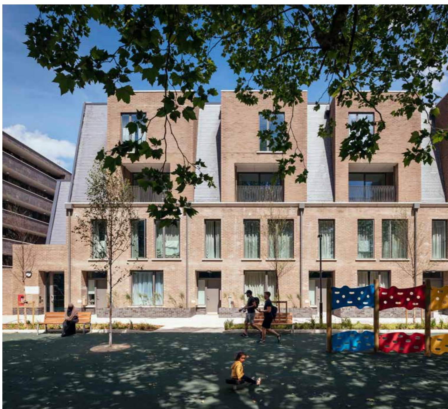
Front view of Block F (Phase 1b), now called 1-15 Hazelbury Way comprising 14 council homes and completed January 2021
