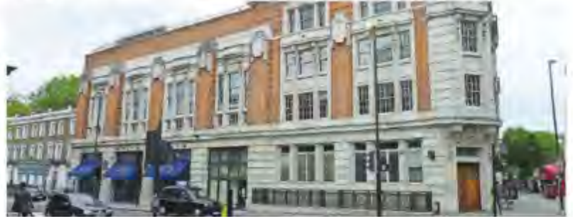
Crowndale Centre is the temporary town hall for Camden.
